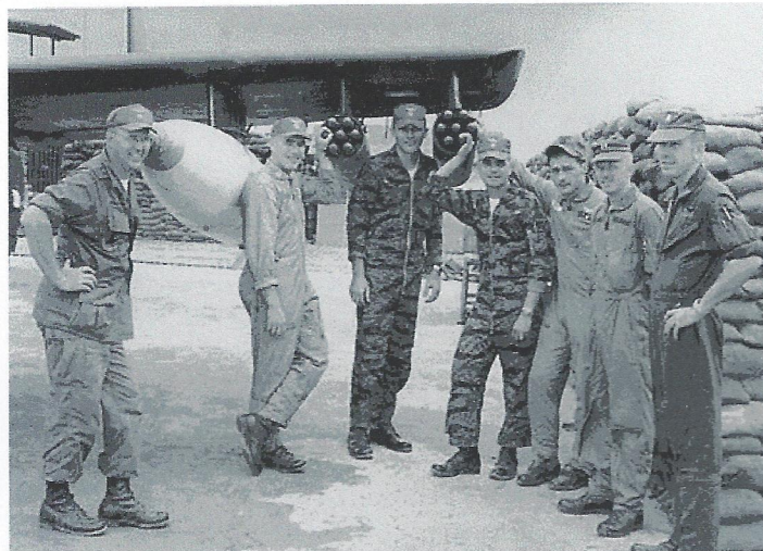
Mohawk shown with two 2.75 inch rocket pods. Normally the inboard hard point had a fifty caliber machine gun installed.
